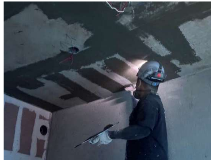
3F天花板批土施作
