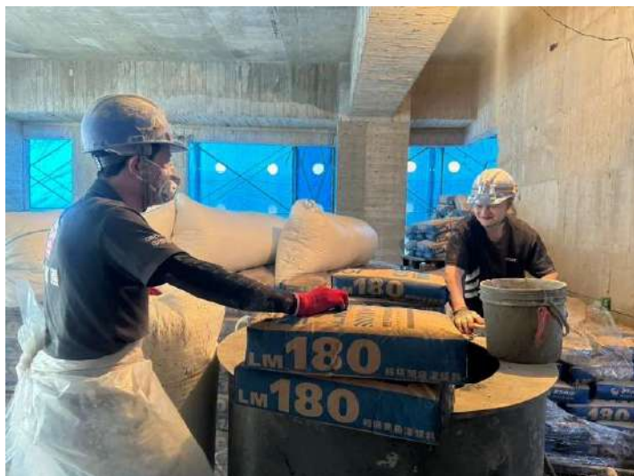
輕隔間灌漿施作
