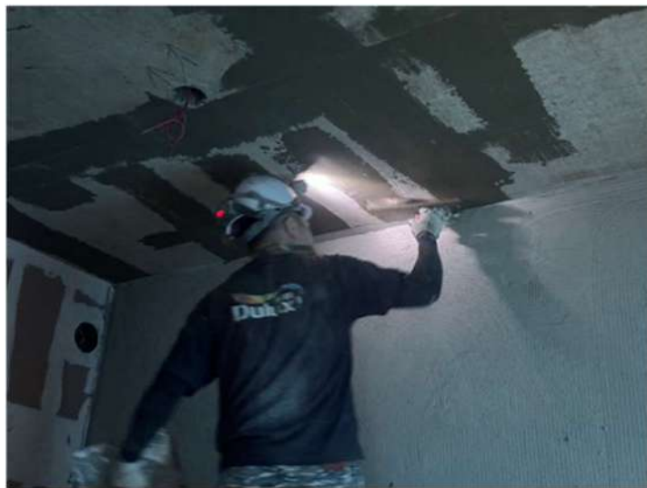
3F天花板批土施作
